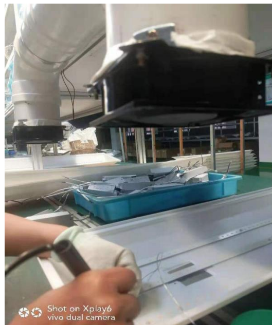
废气收集措施：集气罩
